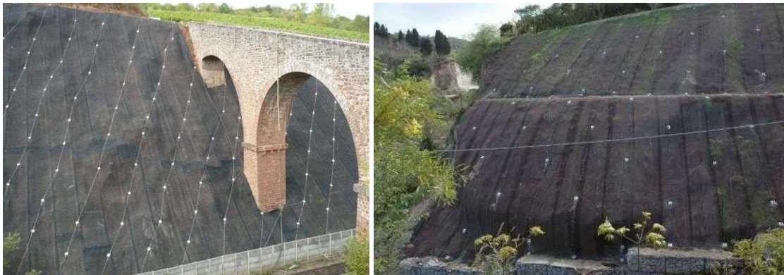
Fig. 2 Soil Nail Wall with Flexible Structural Facia
