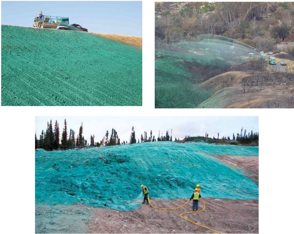
Fig. 5 Application of High Performance-Flexible Growth Medium
